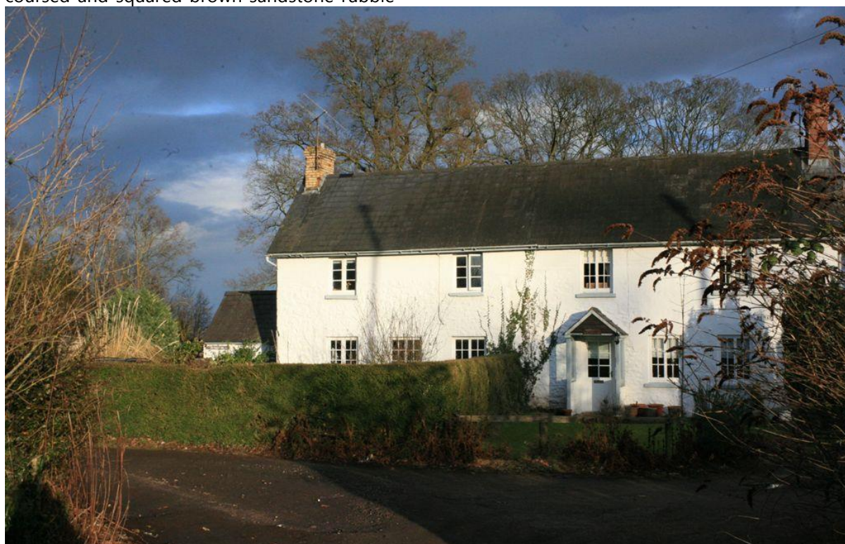
Fig.48 The white painted rubblestone Ty-saar-maen and Ty-saercoed share common characteristics of cottages in Rhyd-y-Meirch (character area 2)
