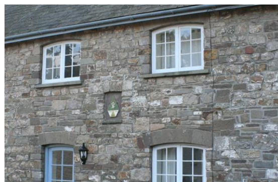
Fig.69 Rubblestone walling is the characteristic material of 19 th century and earlier houses within the Conservation Area
