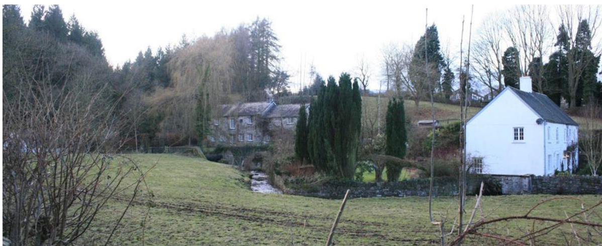
Fig.17 View from Well Cottage to the mill in its valley setting
