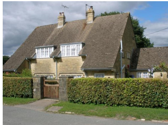
Fig.68 Tre Elidyr. A pair of 1960s cottages infilling a plot in the layout planned by Powell. They contribute to the enclosure of the green and provide street continuity. The form and design of the buildings is a later reinterpretation of the established style of the original houses, although the choice of materials and plan depth of the buildings is less successful.
