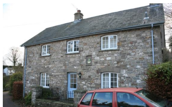
Fig.57 Rhyd-y-Meirch. A larger cottage situated parallel and behind the Post Office Cottages. The skilful use of stone voussoirs forming elliptical arches over the window heads is apparent.
