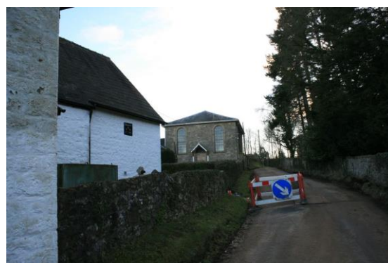
Fig.49 The Hanover Chapel has coursed and squared sandstone rubble walls beside the painted rubblestone Hanover
