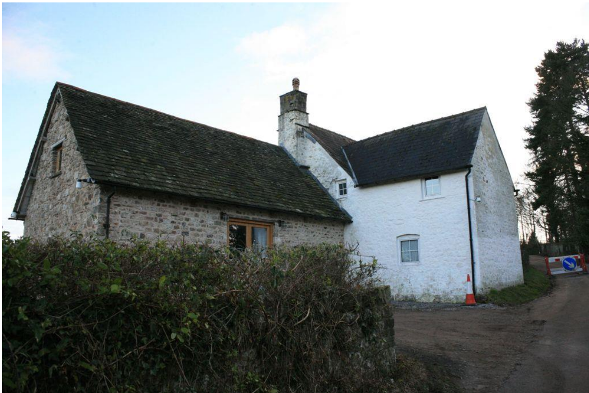
Fig.47 Hanover and attached (converted) barn
