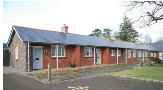
Fig.37 A renovated range (Hall House) forming part of the estate buildings facing a large courtyard; red brick and natural slate roofs
