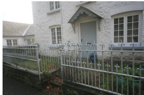
Fig.53 Distinctive historic railings to Y Llyth-yr-dr
