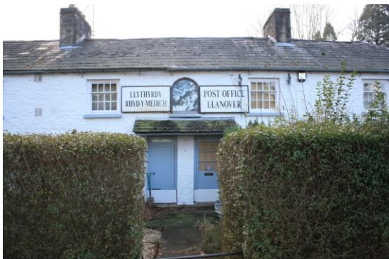
Fig.56 Post Office, Rhyd-y-Meirch. This is part of a regular short terrace dating from the late 18 th /early 19 th century. The plaques with bold lettering are an eye catching feature.
