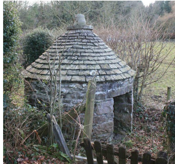
Fig.60 Circular pigsty, restored, in the garden of Well Cottage, Rhyd-y-Meirch. The use of stone in its conical roof is particularly skilful.
