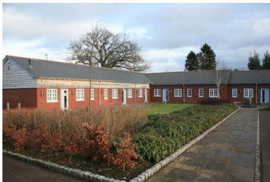
Fig.35 The new Waddington House range making up one side of the Llanover Business Centre
