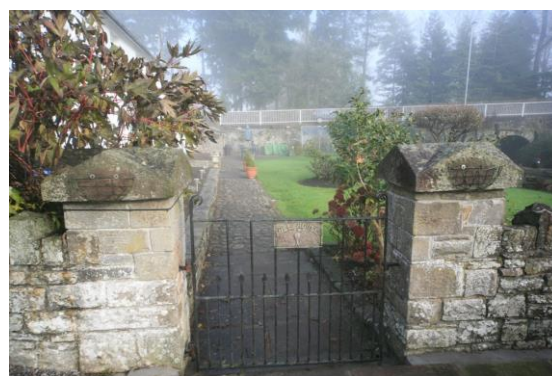
Fig.18 Gate piers to Mill House with unusual capping stones
