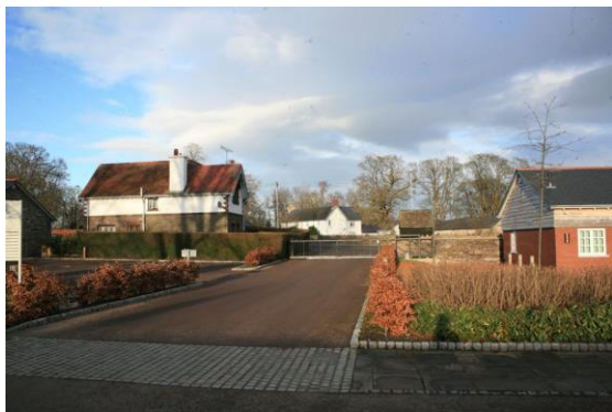
Fig.36 The Police Station with weighbridge and weigh building viewed from within the estate yard. These buildings form part of the important group of buildings which contributed to the management of the Llanover estate.
