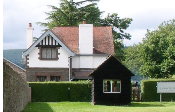
Fig.61 Former Police Station and house, at the entrance to the Llanover Estate Yard. An 'official' and standard design which skilfully uses traditional materials in a robust and attractive design influenced by the Arts and Crafts movement.
