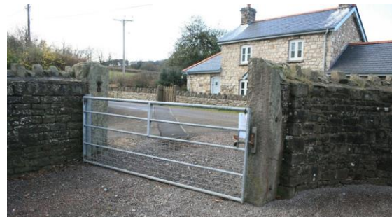
Fig.40 Large rough hewn stone gate piers are a feature of the entrances to the estate yard
