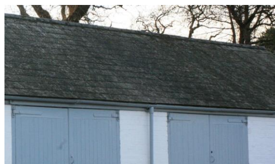
Fig.72 Cement-fibre slates are increasingly seen as natural slate is replaced or on new build
