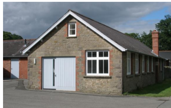
Fig.62 Former Estate Yard building. The logical and sympathetic choice of materials, good proportions and good use of colour, make this group both attractive and functional.
