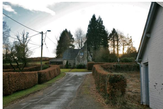
Fig.80 No.5 terminating the view looking south-west along the perimeter road to Tre-Elidyr
